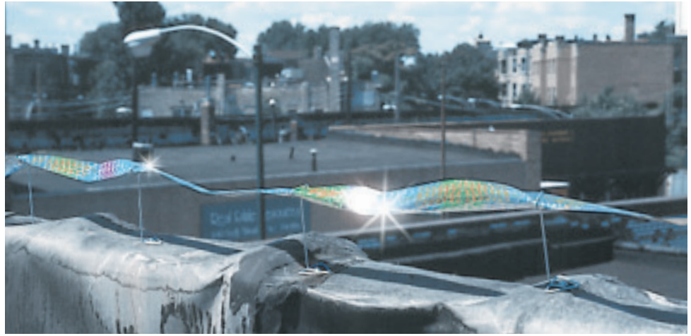
Roof ledges, sills and other linear installations
