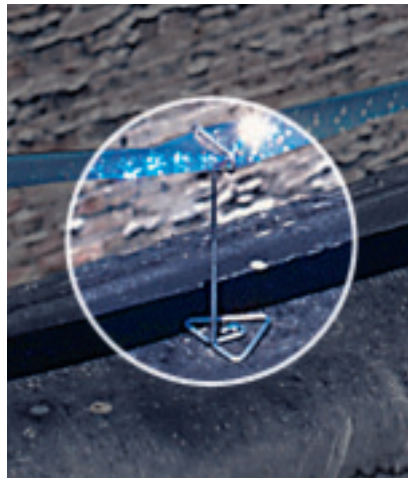
Detail of brackets
